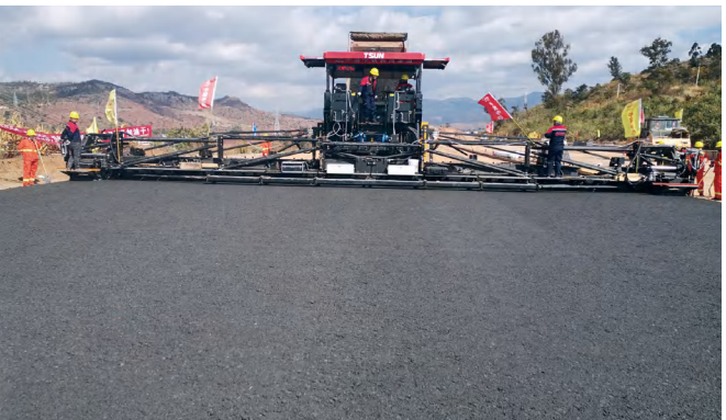
Yuxi-Chuxiong Expressway Paving thickness 35cm
