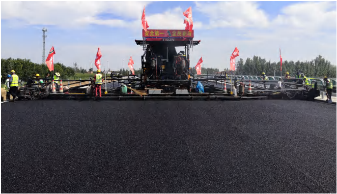
Shandong Section of Beijing-Taipei Expressway Paving width 18.75m
