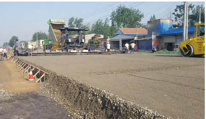
National Highway Paving thickness 50cm
