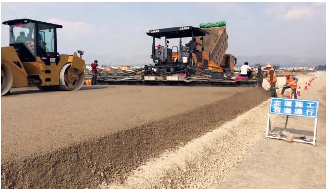
Yunnan Baoshan Outer Ring Road Paving thickness 50cm
