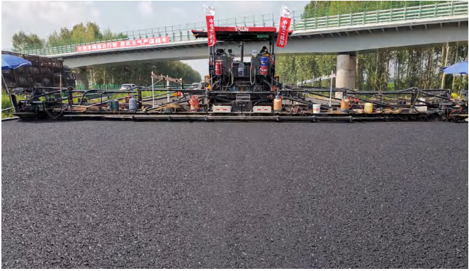
Heilongjiang section of Beijing-Harbin Expressway Paving width 18.75m
