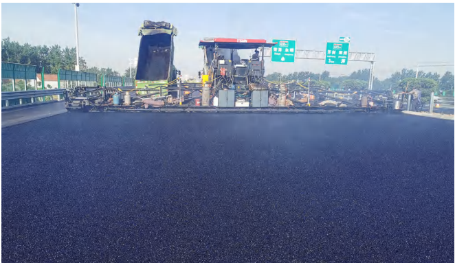
Heze Section of Rizhao-Lanlao Expressway Paving width 18.75m
