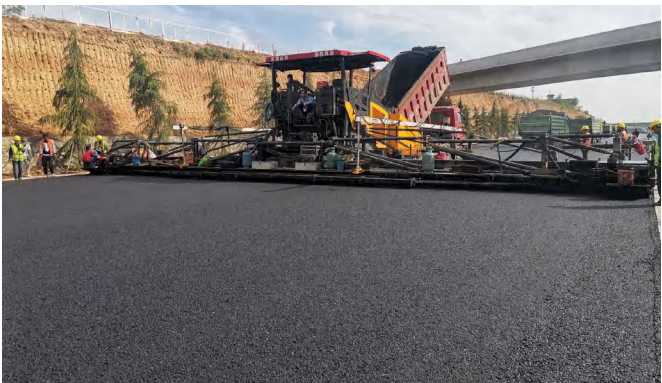
Luoyang section of Erlianhot-Guangzhou Expressway Paving width 18.75m
