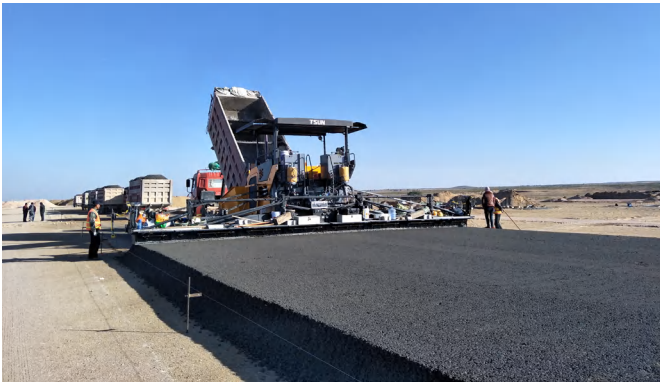
Aodong Expressway Paving thickness 48cm
