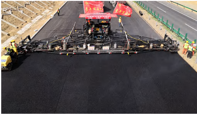
Jilin section of Beijing-Harbin Expressway Paving width 18.75m
