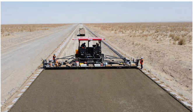
Minfeng-Luopu Expressway Paving thickness 43cm
