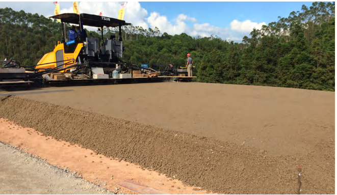
Guigang-Hepu Expressway Paving thickness 48cm
