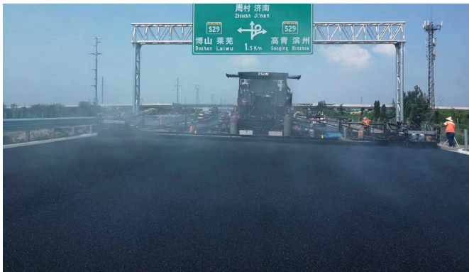
Zibo Section of Jinan-Qingdao Expressway Paving width 18.75m
