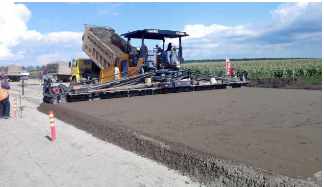
Provincial Road 202 Paving thickness 44cm
