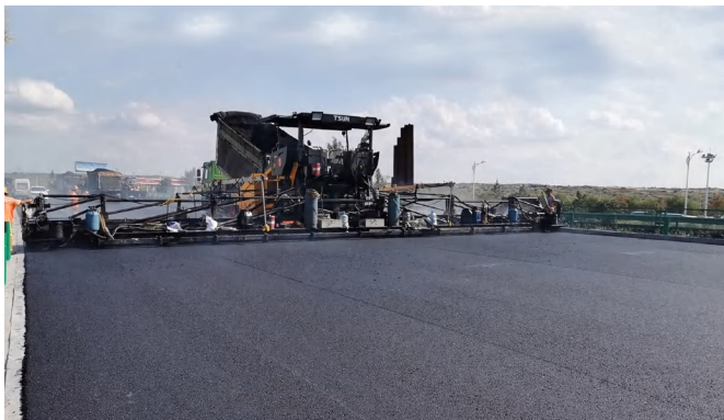
Inner Mongolia Section of Baotou-Maoming Expressway Paving width 18.75m
