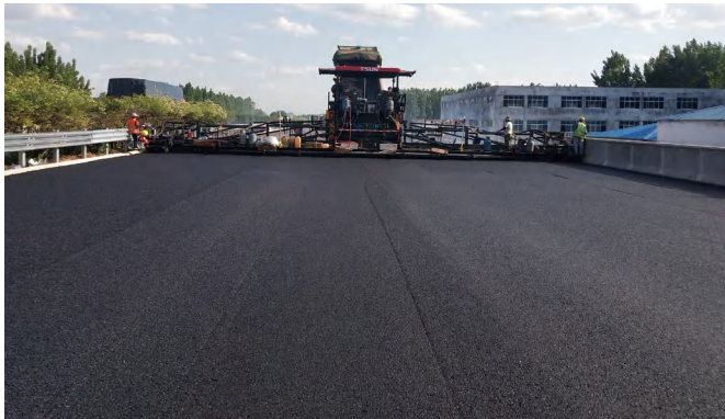
Shandong Section of Beijing-Shanghai Expressway Paving width 18.75m
