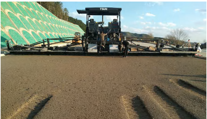
Xundian-Zhanyi Expressway Paving thicnkess 50cm
